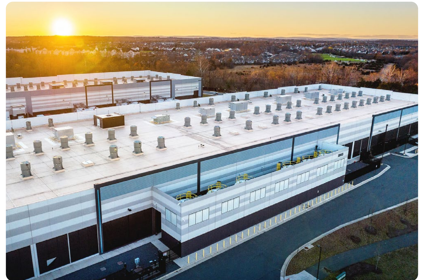
An AWS data center in Northern Virginia.
