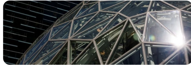
The thousands of panes of glass in The Spheres are designed to maximize light exposure for plants while maintaining a consistent temperature inside.
