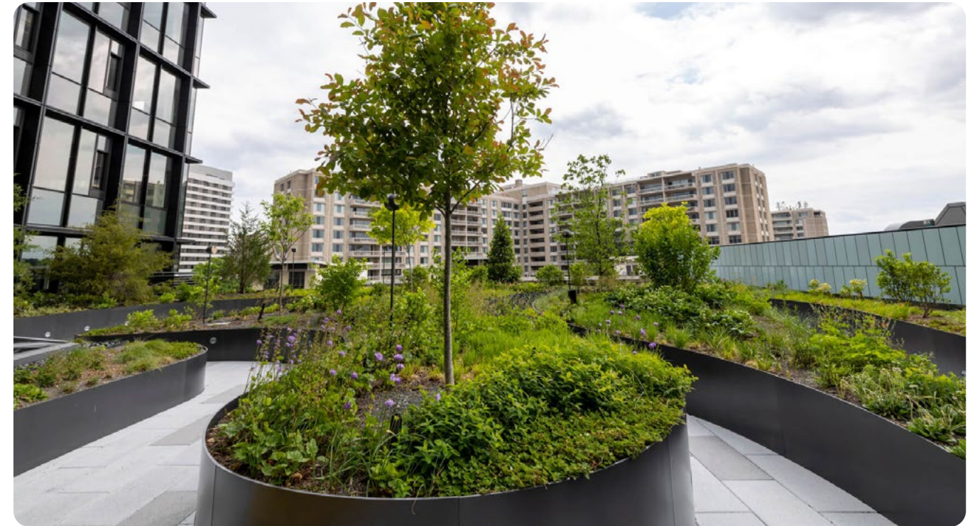
The terrace gardens at our headquarters in Arlington, Virginia, feature recycled greywater systems for irrigation.
