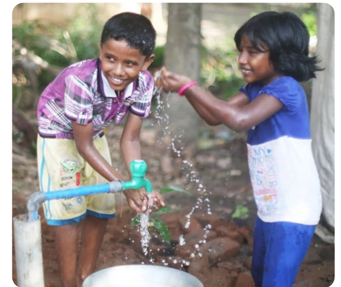
Clean drinking water from an Amazon and Water.org project.
